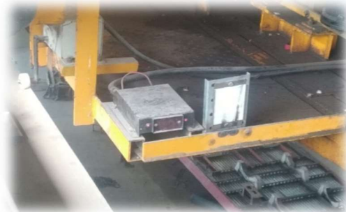
Proximity Sensor installed on Bogie frame machining center
