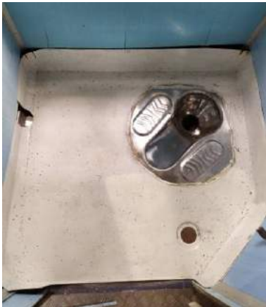
Polysulfide Epoxy Resin Coating Lavatory Flooring
