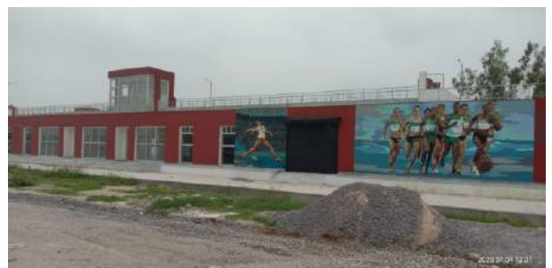
Synthetic Track (Construction work in progress).
