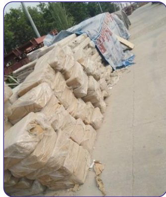
Unloading of Material
